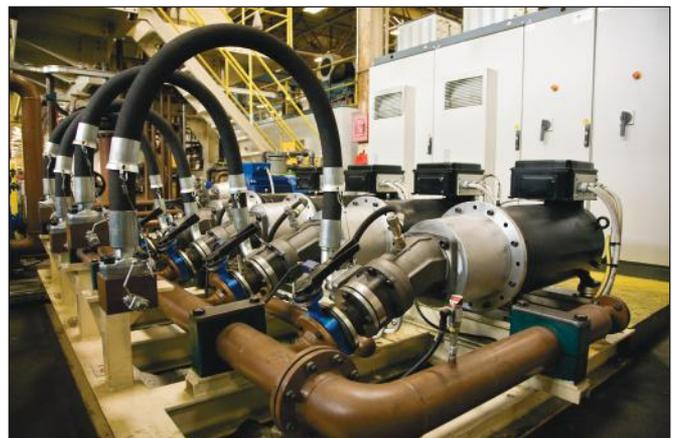
Figure 7. Variable speed hydraulic pumps.
